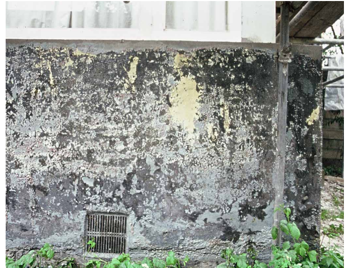
FIG. 2.9 Wall below the kitchen window in the east elevation; B. Mulder chose the dark grey of the top right corner for the new colour scheme
