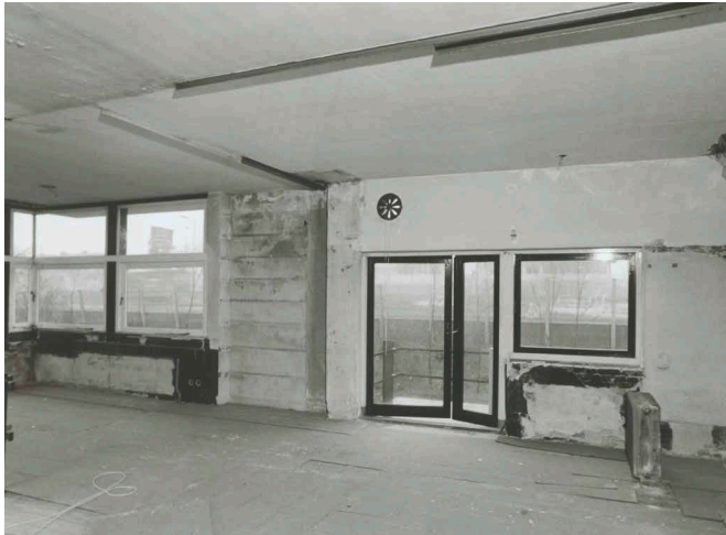
FIG. 3.3 The partially dismantled upper floor
