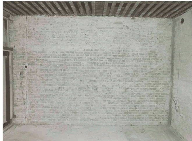
FIG. 3.6 Bare brick wall and stripped ceiling
