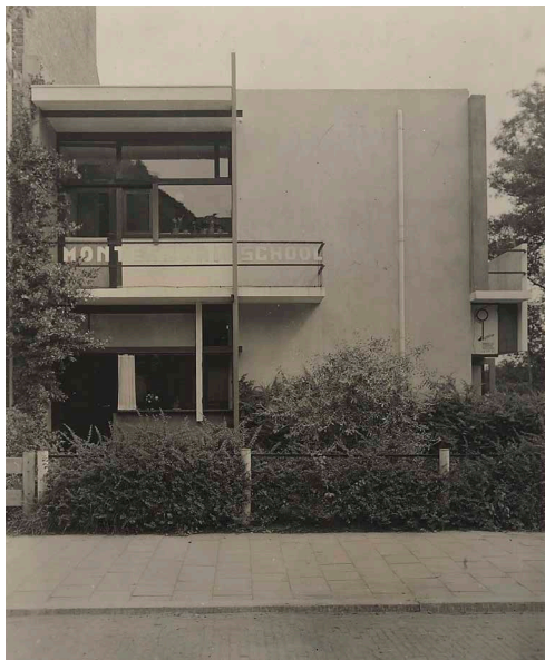
FIG. 2.2 The Schröder House in use as Montessori school, between 1933 and 1936
