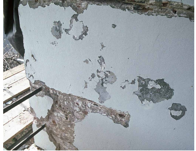
FIG. 2.7 In various places, such as the chimney, B. Mulder found still more finish coats and colours that he could include in his colour research
